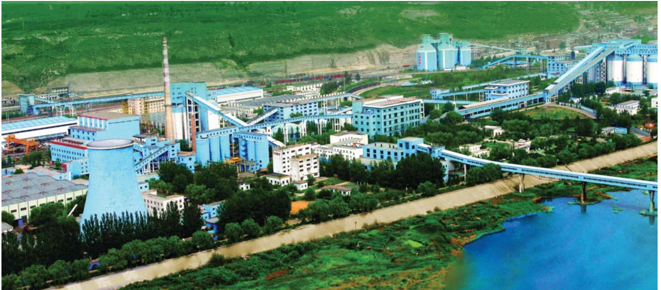
Distributed Underground Reservoirs Have Been Built at the Daliuta Coal Mine in the Shendong Coal Mining Area
