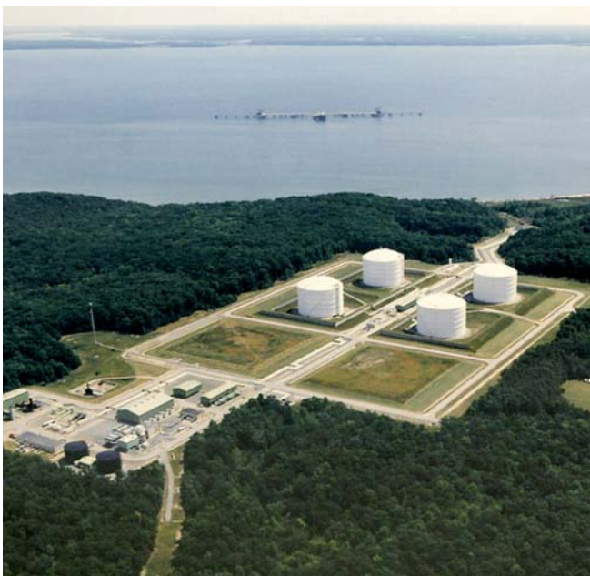
An Aerial Photo of the Dominion Liquefied Natural Gas Facility in Cove Point, Md.
