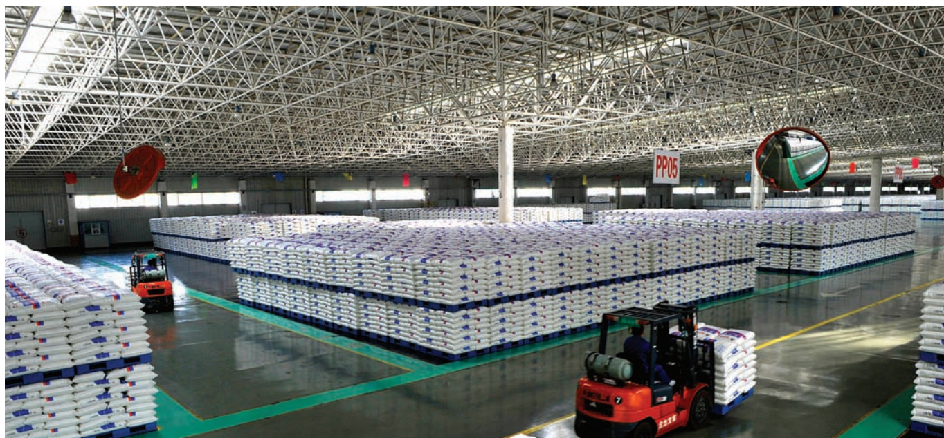
Today the Shenhua Baotou MTO Plant produces 300 ktpa of polypropylene and 300 ktpa of polyethylene.
