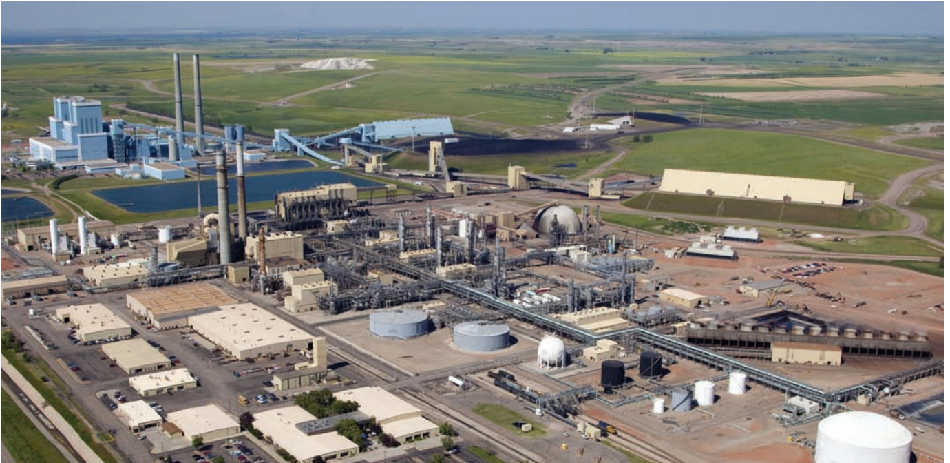
Great Plains SynFuels Plant, operated by Dakota Gas, has been producing natural gas from lignite for over 25 years. Starting in the 1990s, the plant has been selling CO 2 for enhanced oil recovery.
