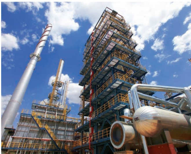
The Shenhua DCL project is the largest DCL project in the world.
