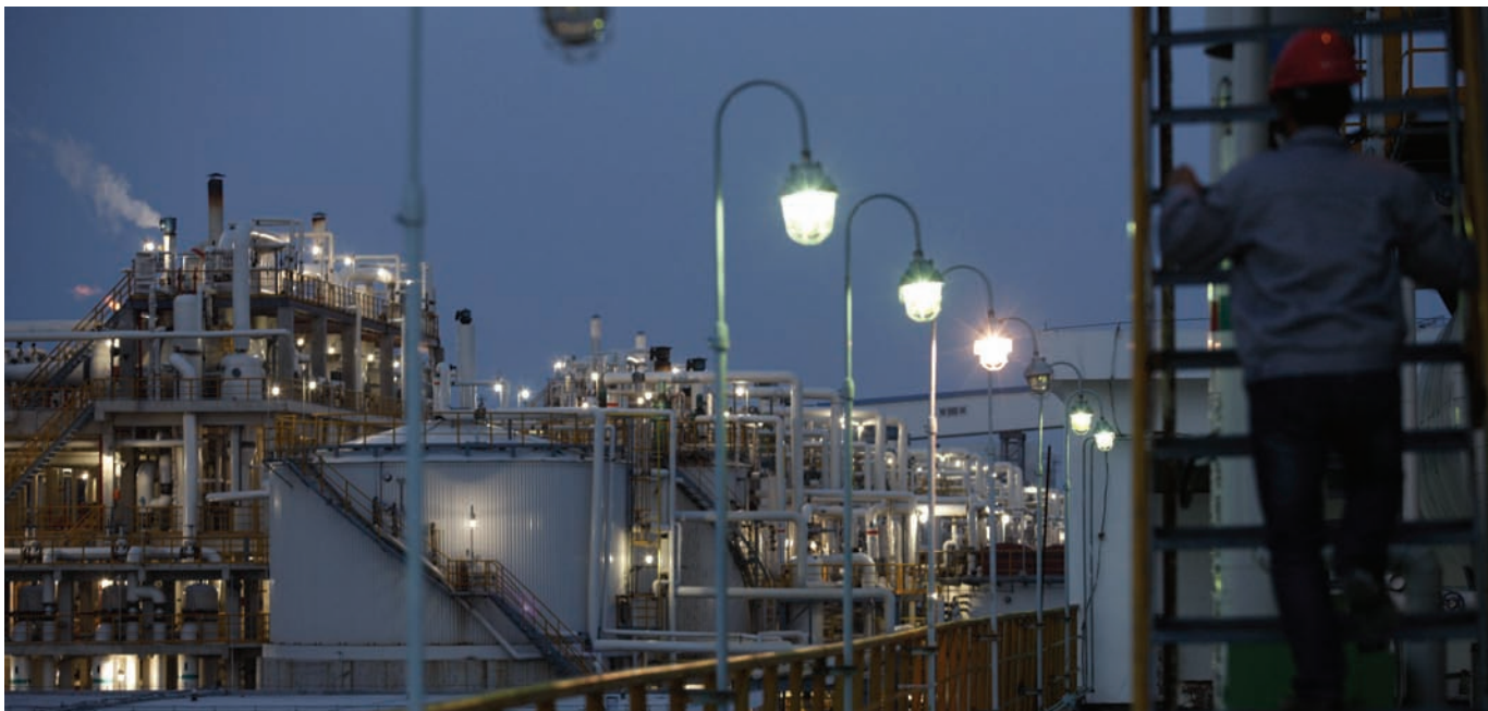
The first production line of the Datang Keqi coal-to-gas facility has been completed and the second line is nearing completion.
