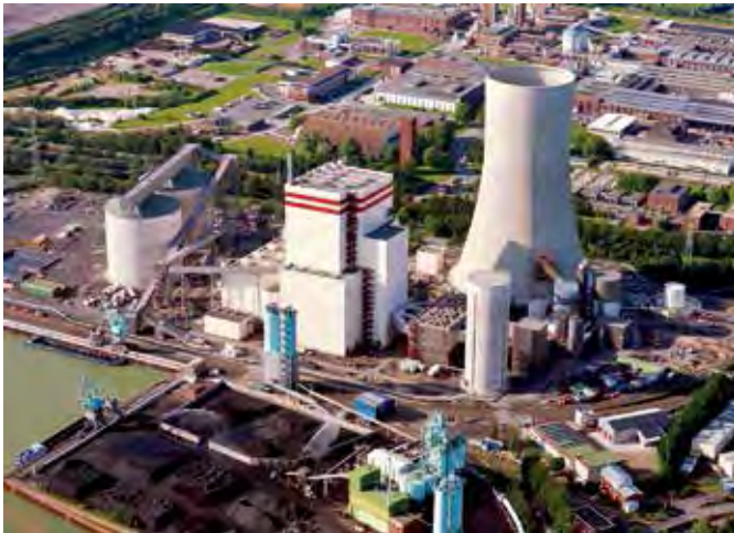
Trianel Kohlekraftwerk Lünen power plant (photo courtesy of Trianel)
