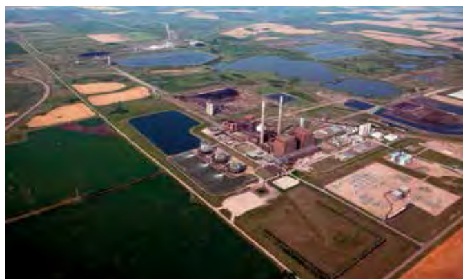
Coal Creek Station has improved performance through coal drying with the DryFining process at both units, in commercial operation since 2009.
