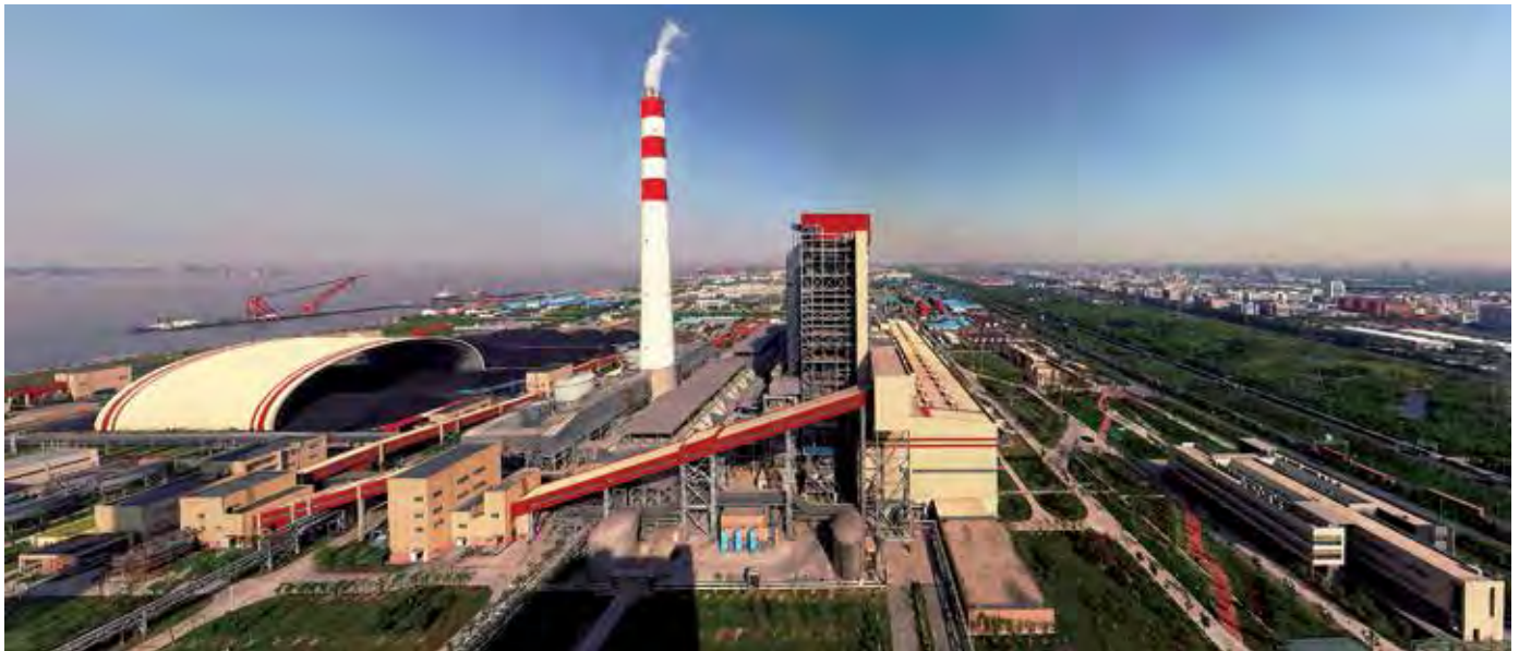
The ultra-supercritical Shanghai Waigaoqiao No. 3 is one of China's flagship high-efficiency, low-emissions coal-fired power plants.
