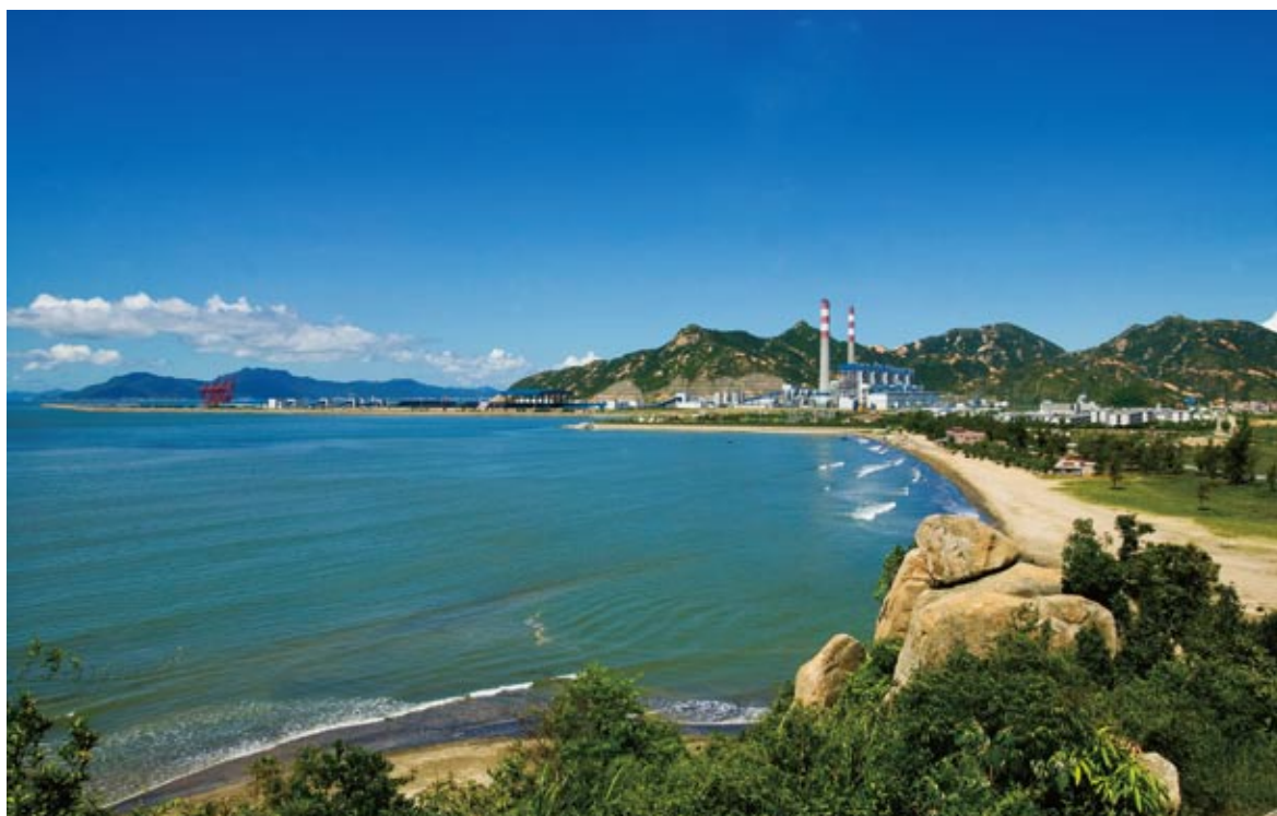
神华国华台山电厂 Shenhua Guohua Taishan Power Plant
