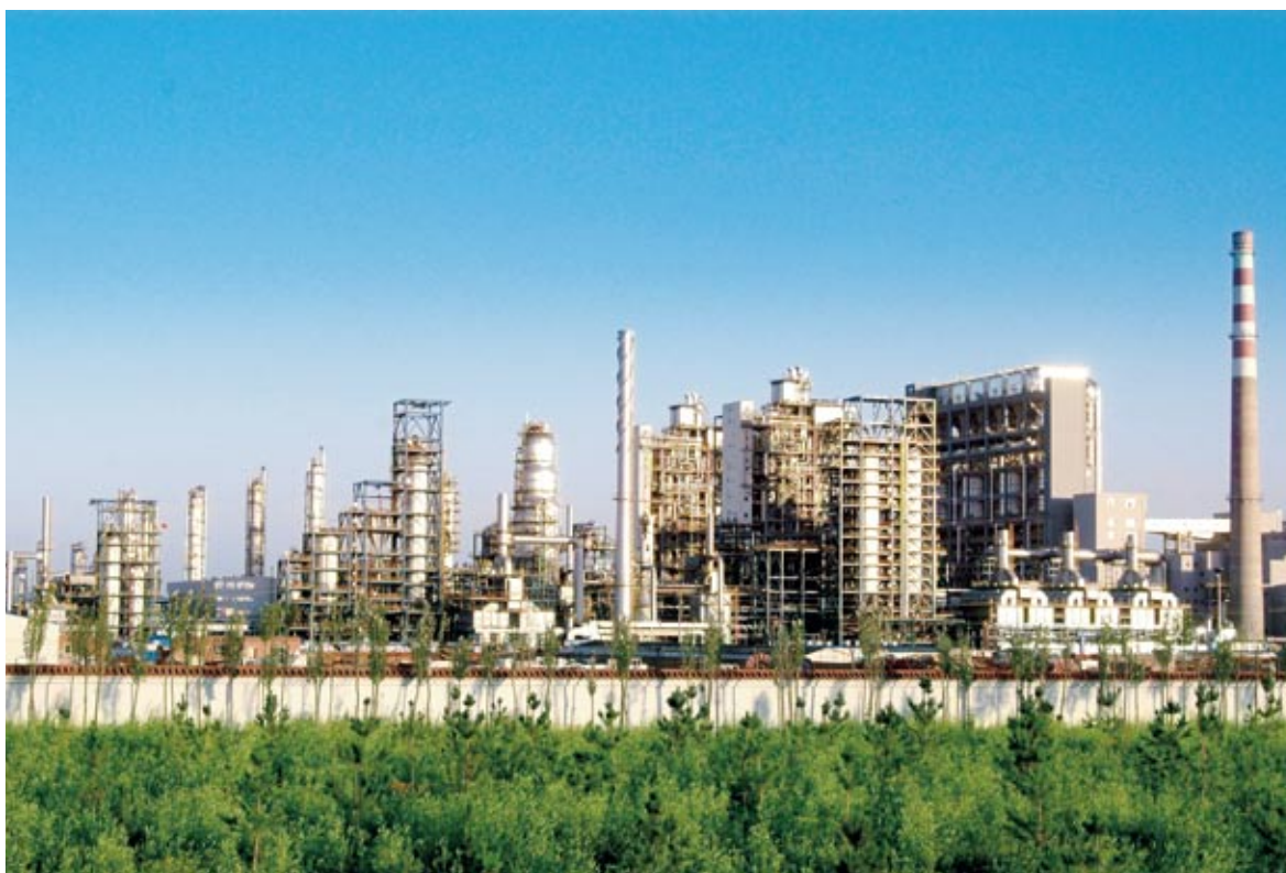
神华包头煤化工分公司生产现场 Production site of Shenhua Baotou Coal to Chemicals Branch
