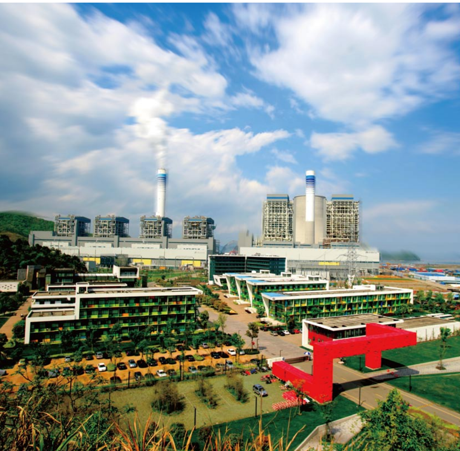
神华宁海电厂全景 Panorama of Shenhua Ninghai Power Plant
