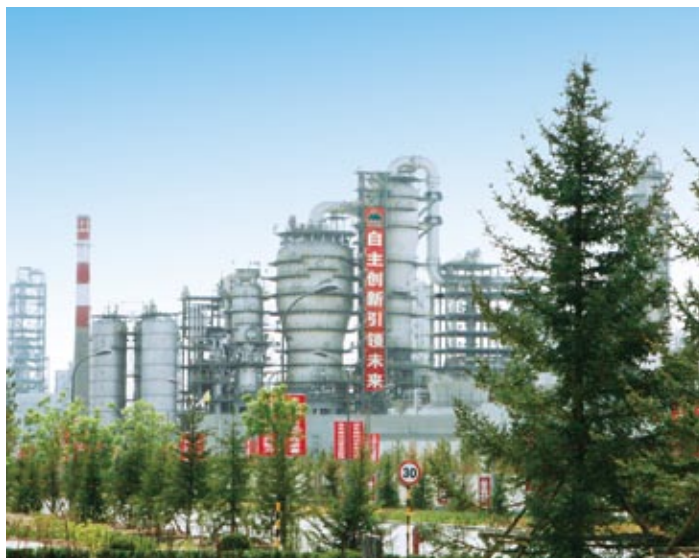
神华包头煤制烯烃项目MTO装置 Shenhua Baotou MTO facility
