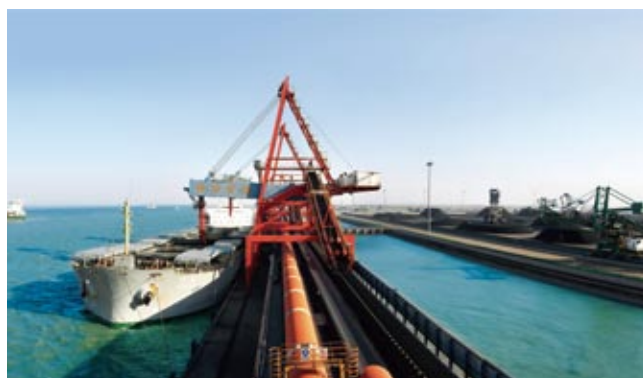
神华天津煤码头 Shenhua Tianjin Coal Dock
